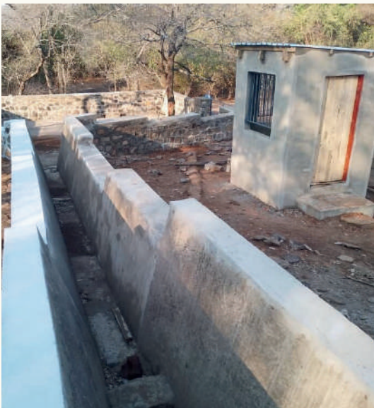
Chitambai dip tank under construction.
