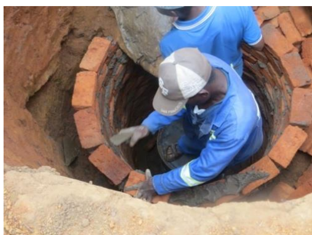
Fig. 12. Sanitation demand in Chimanimani – pit lined with rocks (above), with home made bricks (below) and women being trained in casting the toilet slab
