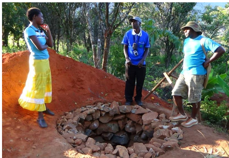
Fig. 12. Sanitation demand in Chimanimani – pit lined with rocks (above), with home made bricks (below) and women being trained in casting the toilet slab
