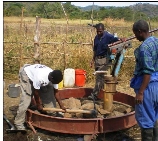
Each of the 15 Village Pump Mechanics had to rehabilitate a borehole before qualifying.
