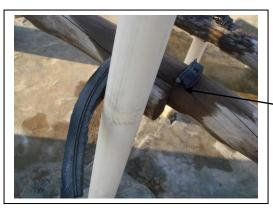
Already a broken strap-support to this 3-month old RWP. Plastic and rubber products tend to deteriorate quite rapidly in the sun as is clearly the case here.
