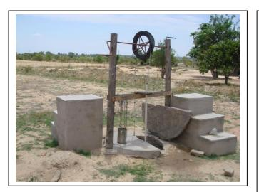
This is yet another example of a RWP that has clearly failed. What was once a perfectly good upgraded family well has now reverted back to being a simple bucket and rope (i.e. no windlass).
