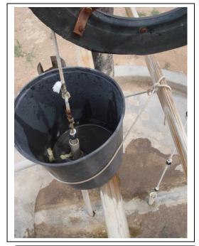
Already significant make-shift repairs have been carried out on this RWP despite recent installation. This is certainly NOT a robust water-lifting device by any measure!
