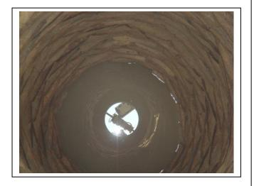
Before being 'upgraded' it is important to ensure that the well will last for many generations. This requires proper lining with burnt clay bricks all the way down.
