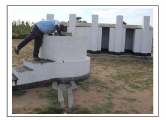
This concrete/brick Hand-Washing Facility (HWF) is far too elaborate and expensive and is in fact not practical. It is neither likely to be filled with water nor properly maintained. The tap is vulnerable and could be stolen and the tank could be vandalised during the school holidays (as has in fact already been reported).
