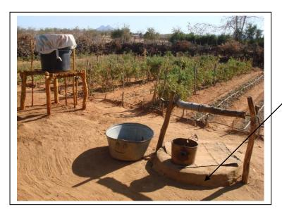
This family could still further upgrade their well ... but it does at least have a sensible if rather basic water lifting device in the form of this home-made timber windlass as well as a tin lid and an up-stand that does provide some form of sanitary seal. The toilet of this homestead is over 30 meters away which is adhering to the general rule: "No well within 30 meters of a pit latrine".
