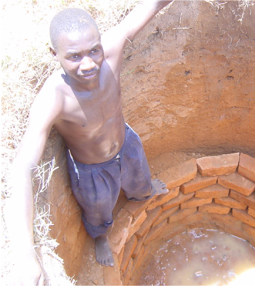
Pits for wells and latrines are lined with interlocking baked clay bricks that fit together without need of cement.
